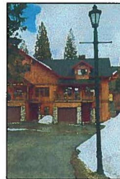
Roof dormers create interesting forms
