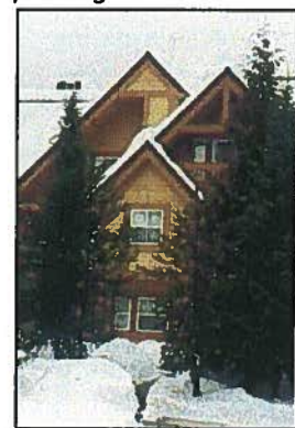
Integrate with the existing landscape features of the site.
