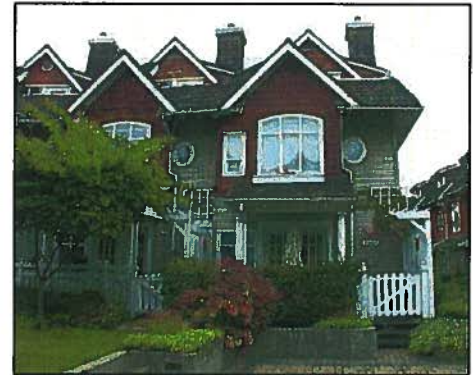
Use colour to accent building elements
