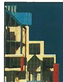
Dropping down towards the lower buildings.
