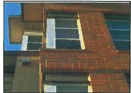
Brickwork emphasizes windows
