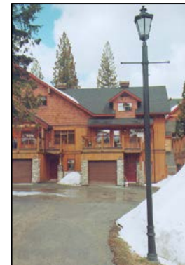
Roof dormers create interesting forms
