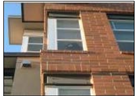
Brickwork emphasizes windows
