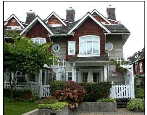
Use colour to accent building elements
