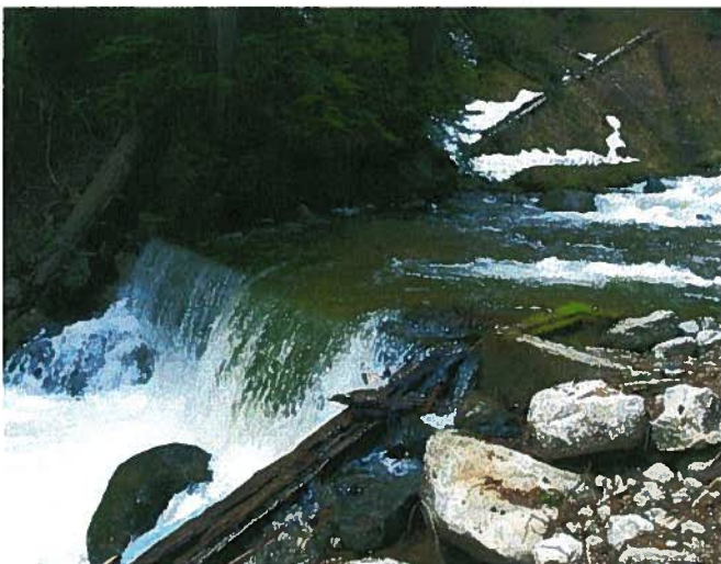
Hanna Creek Raw Water Intake
