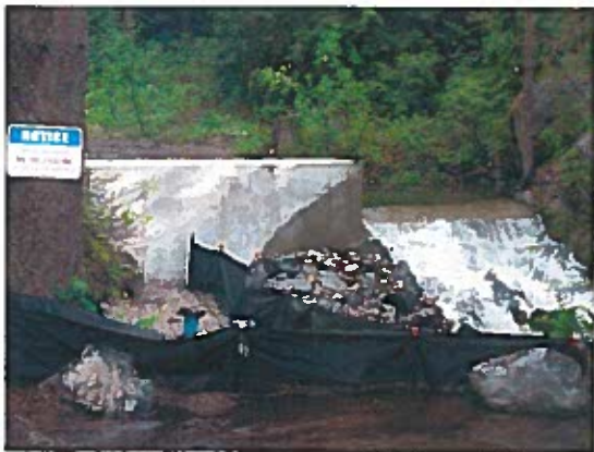
Topping Creek Raw Water Intake
